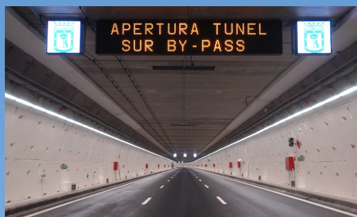
M30 South Bypass Tunnel. Madrid.
